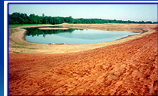
1993: After excavating soil, the west field was graded and seeded to support wetlands.
